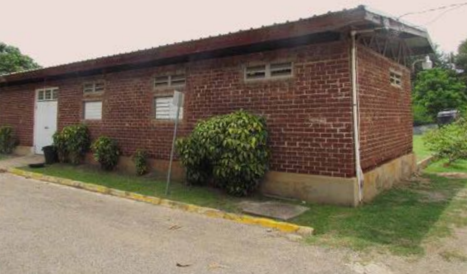
Construction using bricks made from residue
