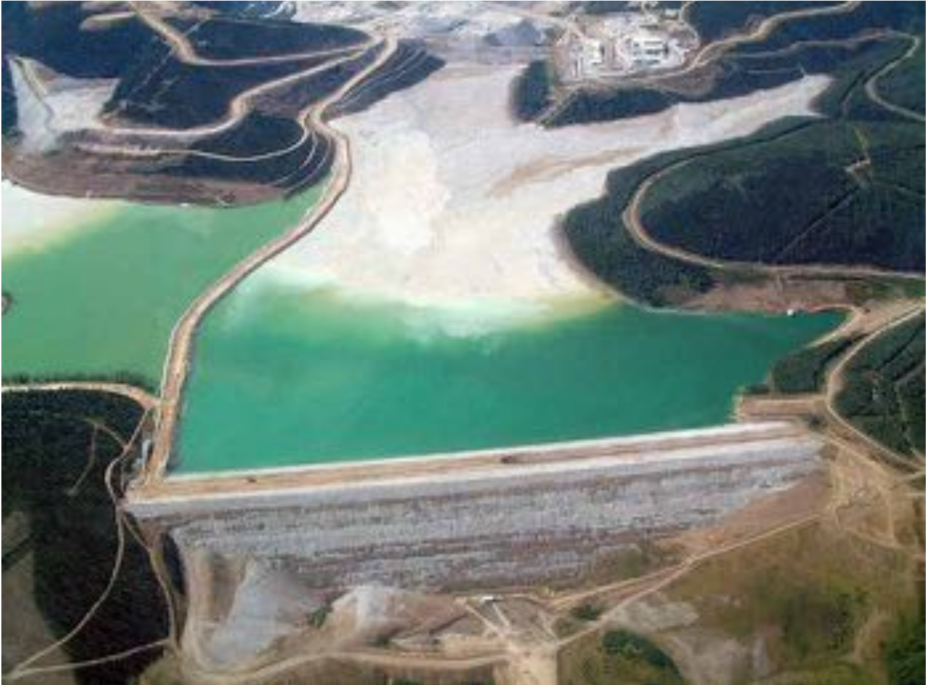
Example of a tailings dam/storage facility – The Fort Knox gold mine in Alaska. The tailings are contained in a valley behind an earth and rock embankment that creates a dam. This tailings storage facility is eventually expected to cover 395 hectares and store approximately 270 million tonnes of tailings (calculated as equivalent dry weight, Kinross Gold Corporation 2015).
